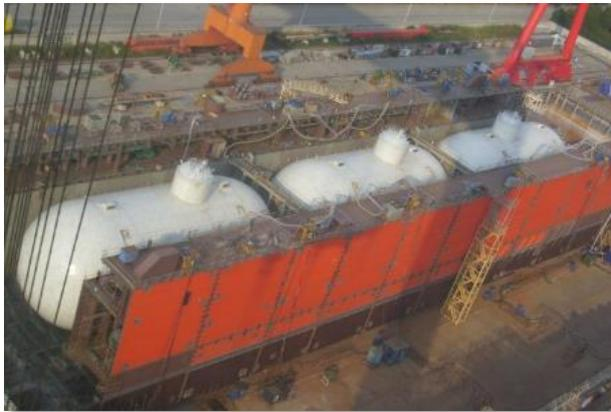
*Type C cargo tank installation on a FLNG*
